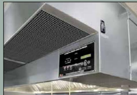
With our commitment to green energy savings, Hood Depot™ offers the Demand control panel, a hood controller with logic circuit that adjusts fan speeds according to peak and slow cooking times to save energy --and money.
