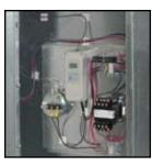
Control panel includes motor starter, control transformer, disconnect switch and distribution block.
